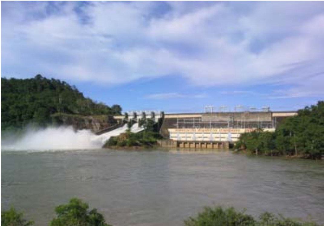
Photo -3-1 Exterior View of Nam Ngum Hydropower Plant
