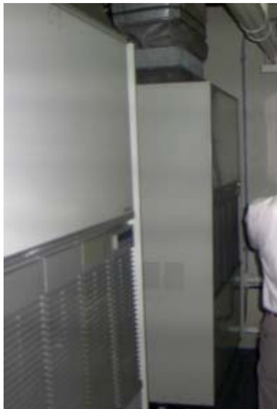
Figure V-4-4 Water Cooled Packaged Air Conditioner
