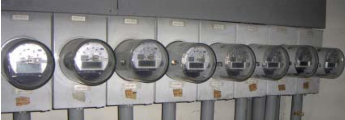
Figure V-4-2 Watt-Hour Meters
