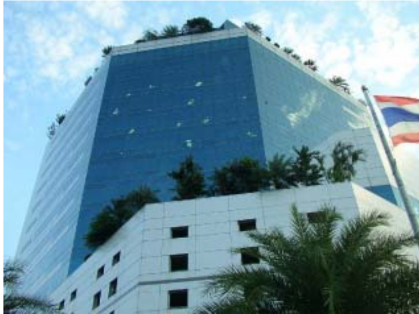
Figure IV-3-1 EGCO TOWER Appearance
