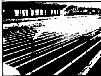
Fig-7 Water being sprayed over roof
