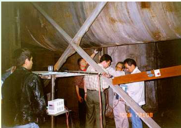
Steel works audit (Blower performance check)
