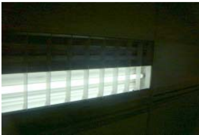
Figure V-4-5 Two-Lamp Fluorescent Lighting with One Lamp Off
