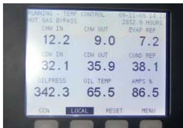
Photograph 3.5 - 1 Chiller Panel Display
