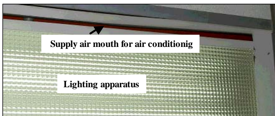
Photo 2.1-3 Lighting apparatus and air conditioner supply air mouth
