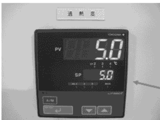
Photo 3 Superheating Degree Indicator
