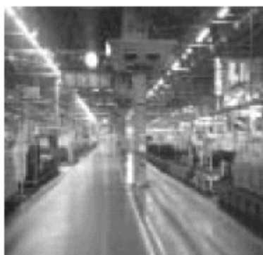
(Fig. 17) The Aisle to which AC-04 Unit was Sending Air
