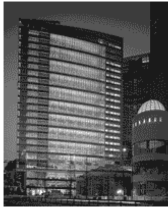
Fig.1 Overview of the target facility
