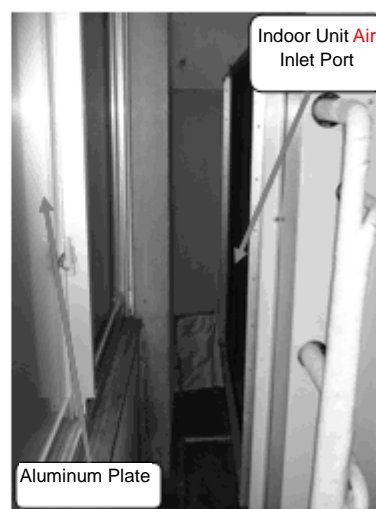
Fig. 17 Aluminum Plate behind Inlet Port
