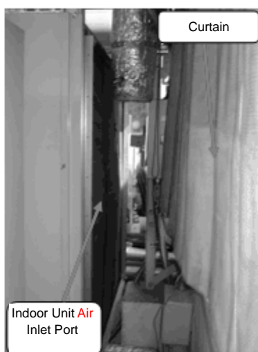
Fig. 16 Curtain behind Inlet Port
