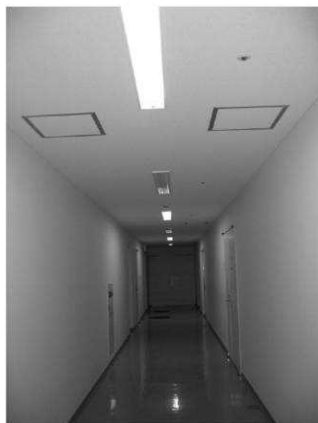
Fig. 5 Thinning out a Lighting in the Corridor
