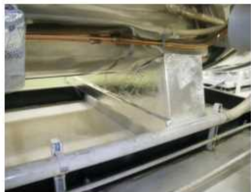
Photo-16 After thermal insulation of boiler legs
