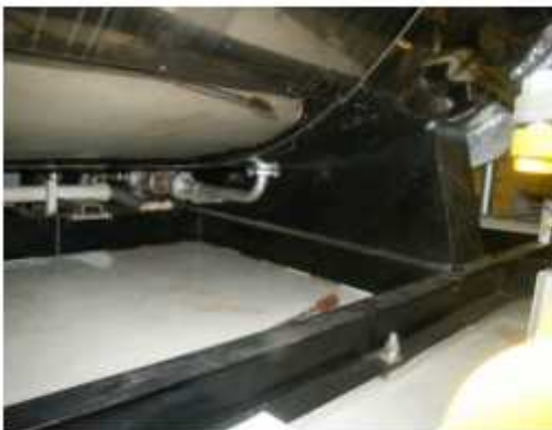
Photo-15 Before thermal insulation of boiler legs
