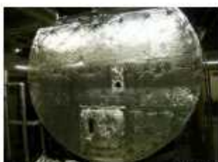
Photo-11 After thermal insulation of boiler mirror plate
