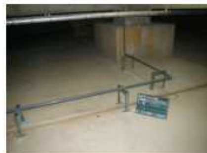
Photo-10 After drain piping repair
