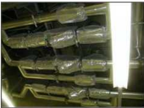
Photo-13 After thermal insulation of steam valve
