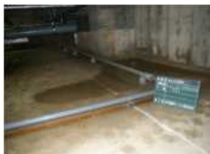
Photo-8 After drain piping repair
