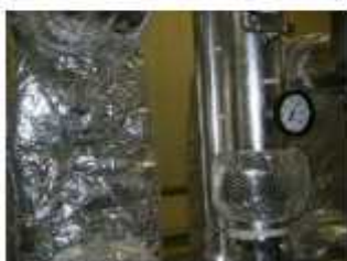
Photo-12 After thermal insulation of plate heat exchanger
