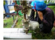
Steam Trap for L.P. Steam Transfer Line (Reflow-made, 1" Free Float Type)
