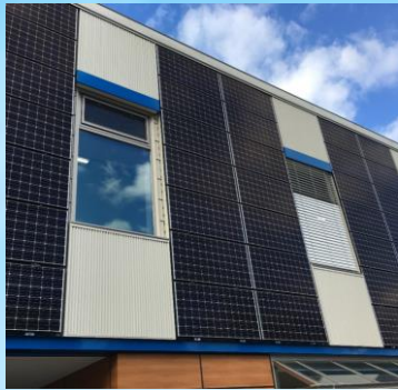
Wall Solar Panels and Low-e glasses windows
