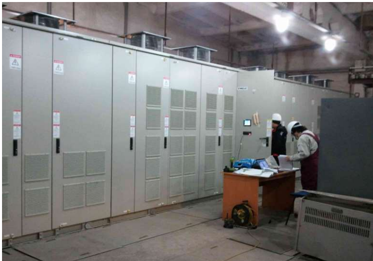
Water pump drive system in Kazakhstan (11kV/2650kVA MVG2)
