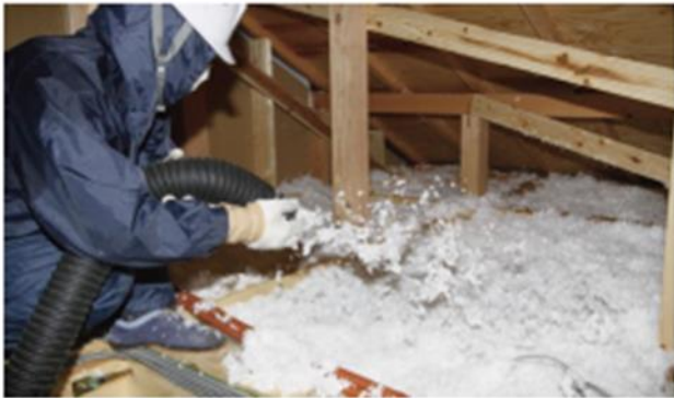
Above the ceiling
