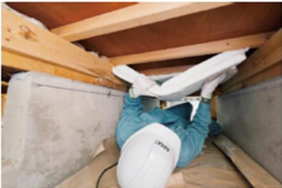
Under the floor
