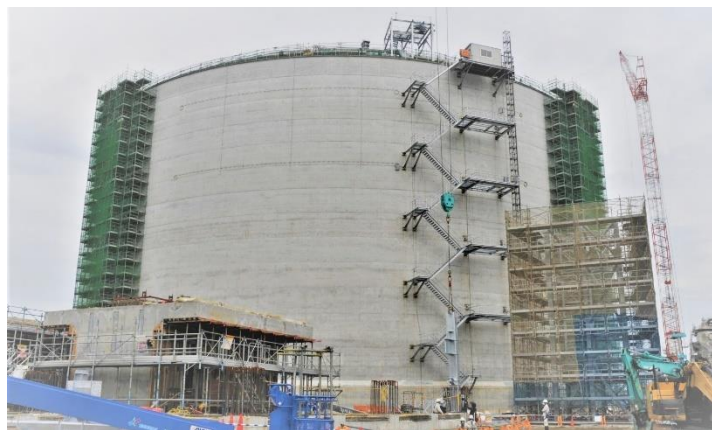
Building an LNG tank, the largest of its kind in Japan, on the premises of Ehime Works
