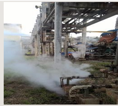
Steam leakage
