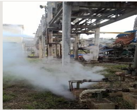
Steam leakage
