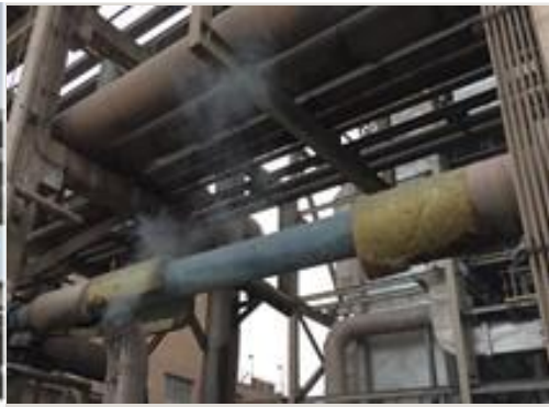
Broken insulation
