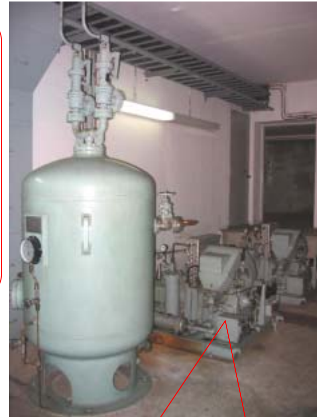
Air Compressor for Governors of Unit No. 1, 2, 3, 4 & 5
