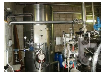
Figure 2: Hot water tank
